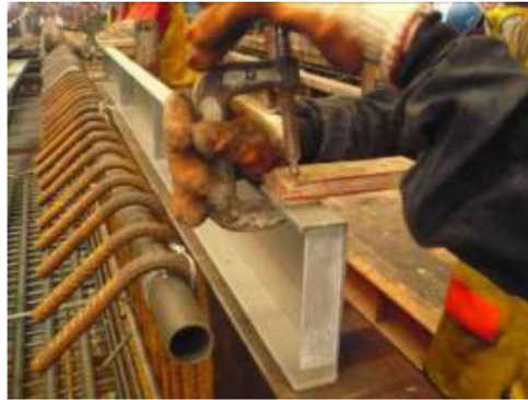
Laying of embedded parts
