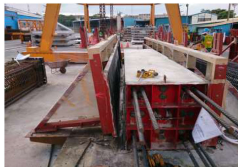
Removal of all related molds
