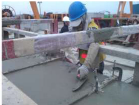
Concrete surface whitewashing
