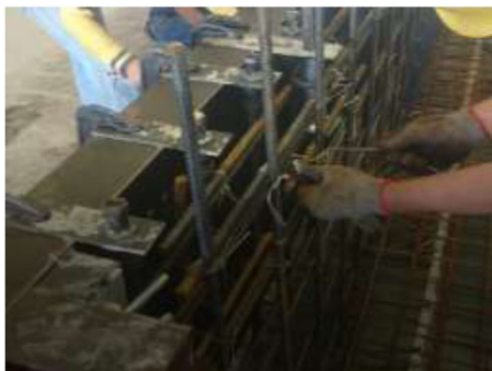
External-wall reserved reinforcement
