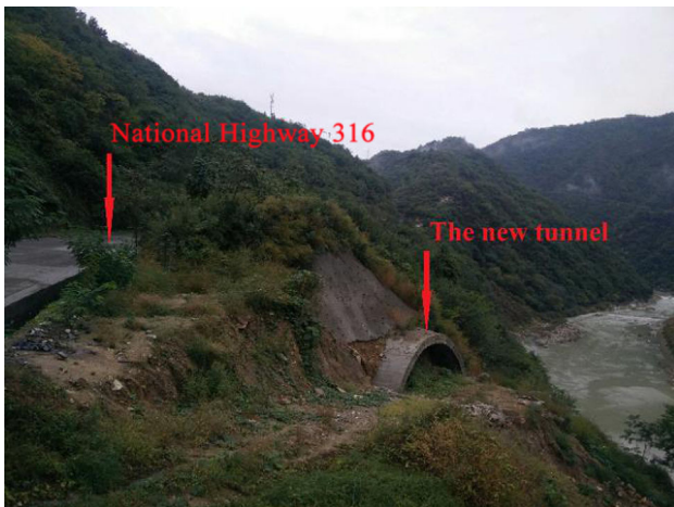
Fig. 3 Actual situation of the new tunnel under National Highway 316
