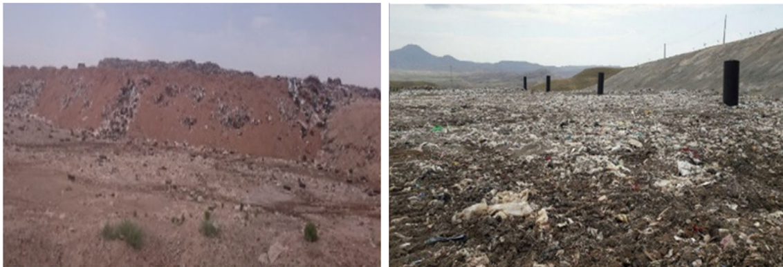
Fig. 2 A view of old (left) and new (right) pictures of the Tabriz landfill
