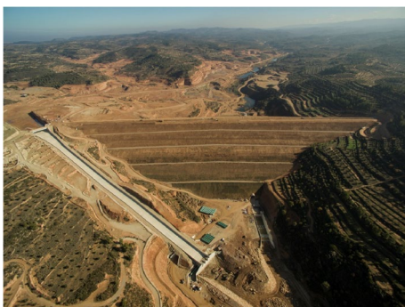
Fig. 1 Albagés dam in May 2017
