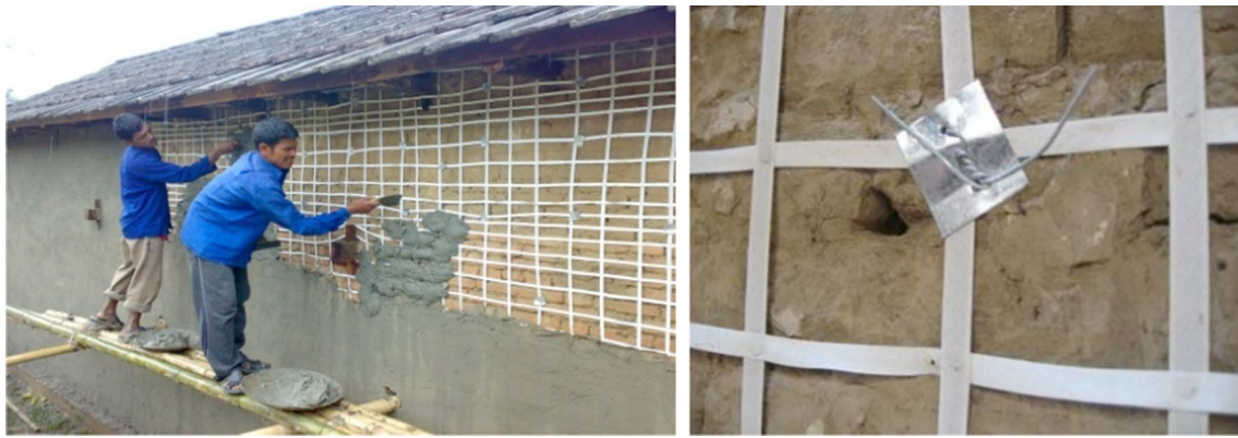
Fig. 22 Implementation of the PP band method of retrofitting in Kathmandu Valley (left) and anchorage throughout the wall (right) (Adopted from Shrestha et al. 2012)
