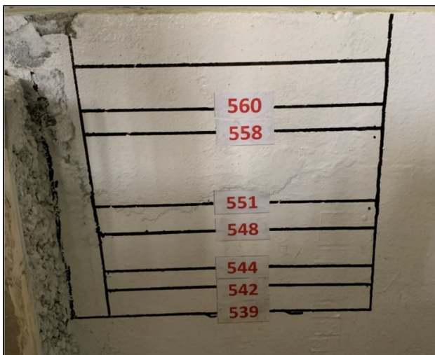
Fig. 5 Reservoir levels marked on the inside wall of the tank
