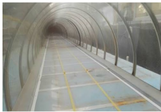
a Lane separation line and curb
