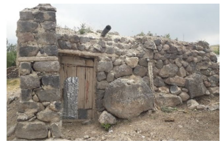
(c) Random rubble masonry wall
