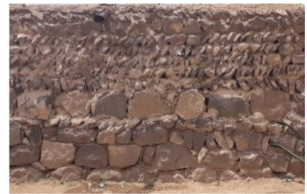
(f) Mixed style masonry wall (Coursed-random bottom and herringbone top)
