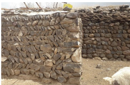
(a) Herringbone and coursed rubble masonry walls
