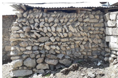
(b) Herringbone rubble masonry wall
