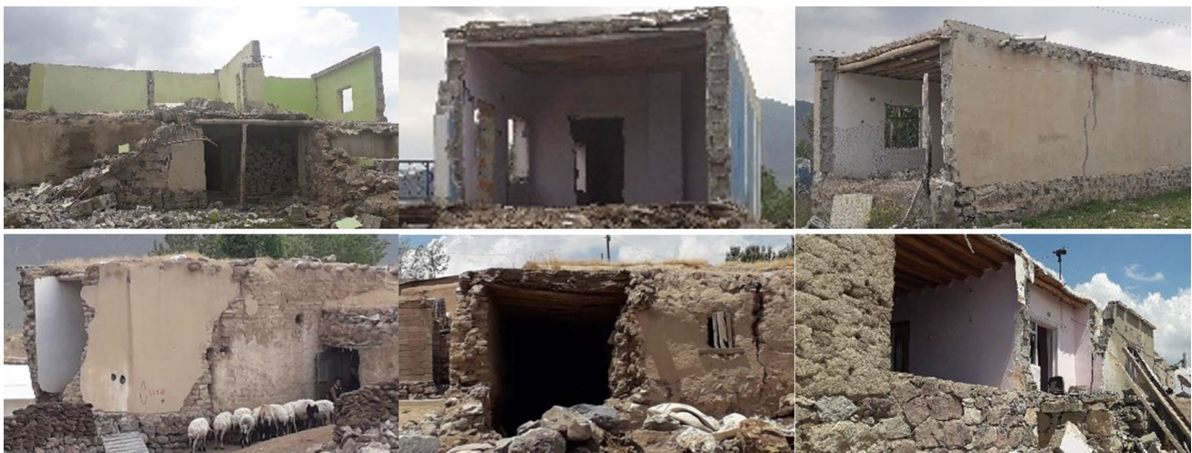
Fig. 14 Out-of-plane failures
