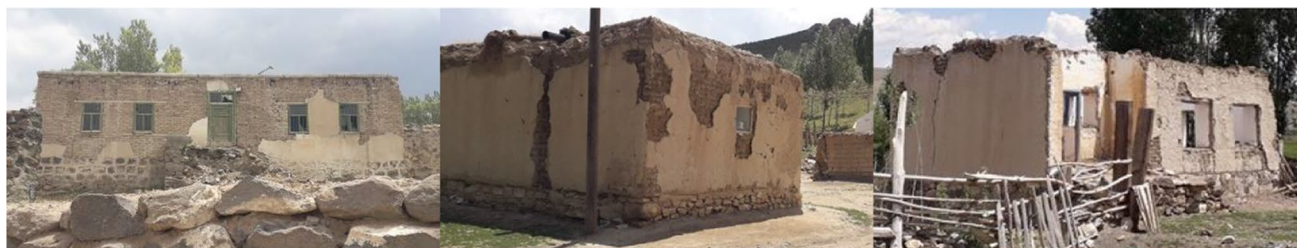
Fig. 21 Well behaved old adobe buildings
