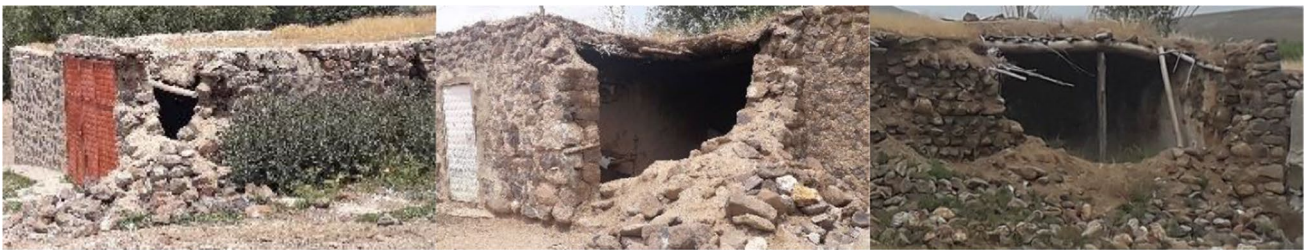
Fig. 15 Corner failures
