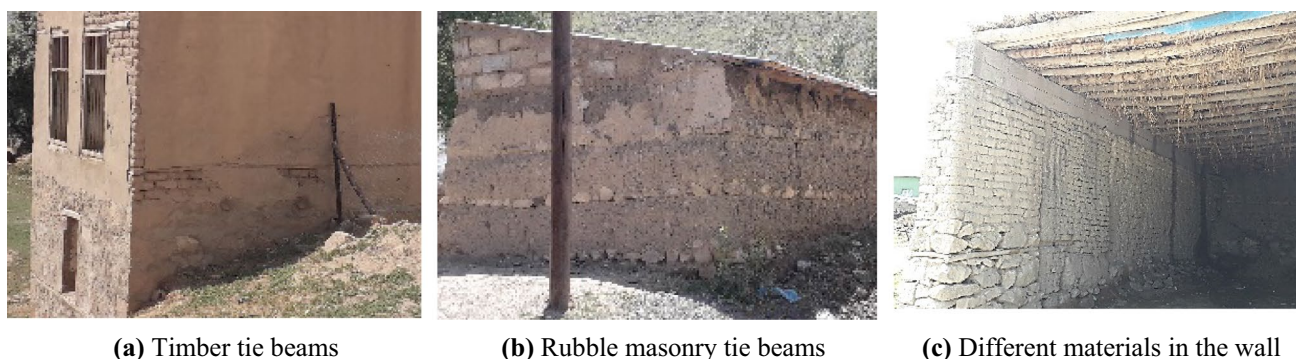
Fig. 6 Different tie beams and wall materials
