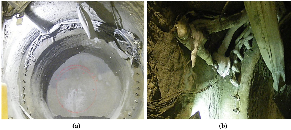
Fig. 1 Freezing technique to provide excavation support for the tunnel (Metro Line 4-Budapest)
