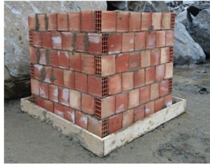
(c) The photograph of constructed masonry wall
