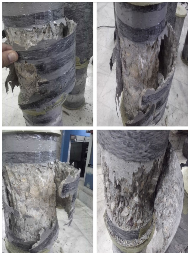
Fig. 10 Example failure modes of discontinuously CFRP-confined concrete specimens
