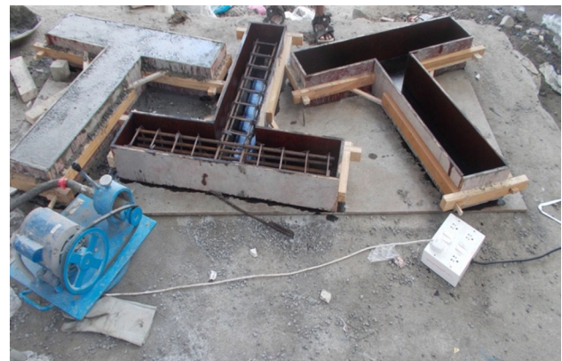
Fig. 3 Form work arrangements and casting work
