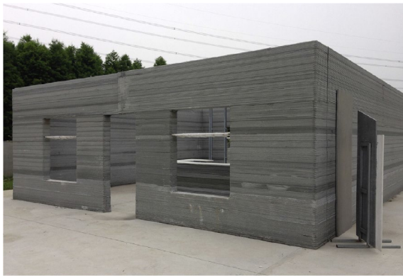
Fig. 20 Winsun building structure developed using AM [15]
