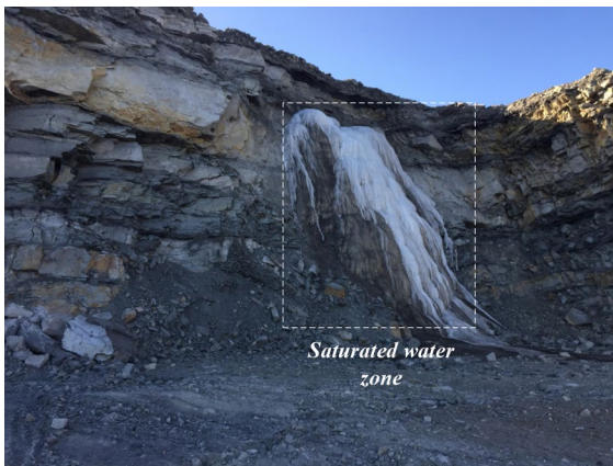
Fig. 2 Characteristics of frozen rock-soil mass around the open-pit mine slope spring
