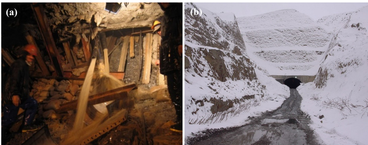
Fig. 4 a Difficulties in tunnel construction due to water adjacent faults 9 and 10 b high precipitation levels in areas near the tunnel
