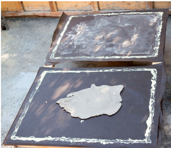
Fig. 8 The membrane walls of the grouting assembly
