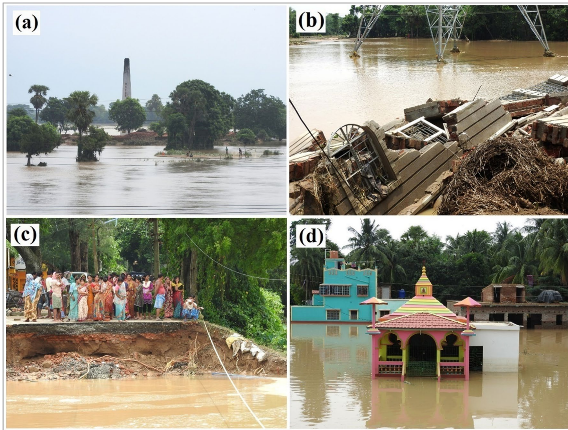
Fig. 17 a Flood inundation of road and agricultural land at Heta-mChak village of Pursurah C.D. block, b house collapsed by flood water flow at Ghola village of Udaynarayanpur C.D. block, c part
