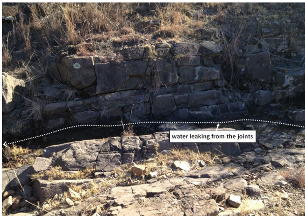
Fig. 8 A dolerite sill exposure with an abundance of orthogonal joints and shear fractures from which water was continuously leaks at the time of observation
