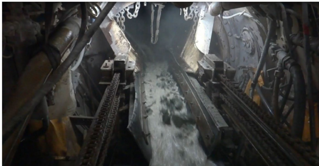
Fig. 23 Actual values of water inflow into the tunnel in the southern portal and water inrush into the tunnel
