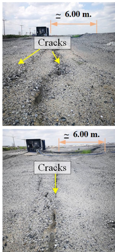
Fig. 11 Photographs of the ground cracks in Zone 3
