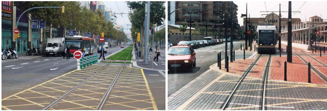
Fig. 5 Road carriageway near an intersection with a tramway line (Spain) [7]
