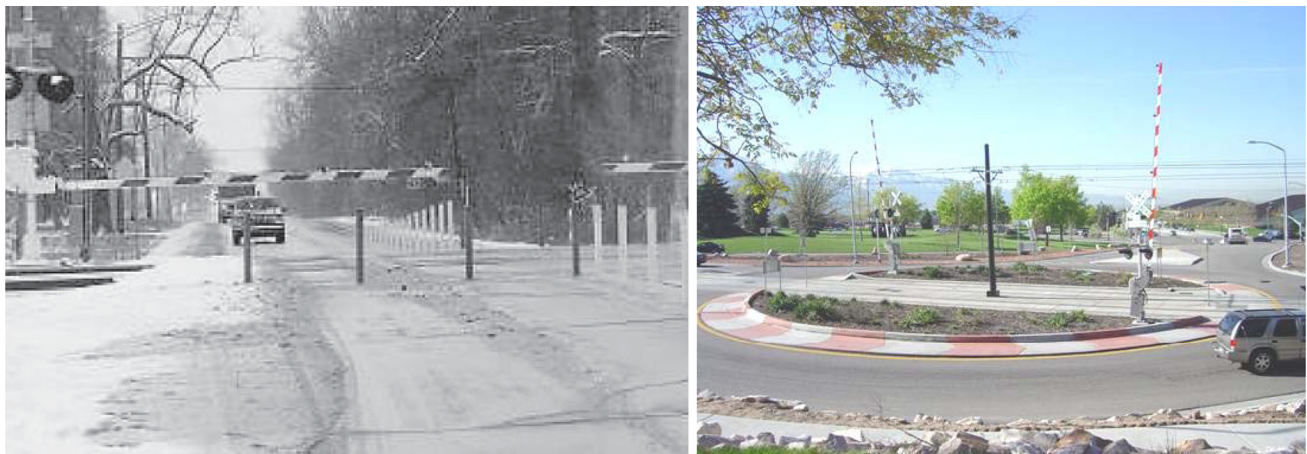
Fig. 7 Barrier installations at at-grade and roundabout intersections
