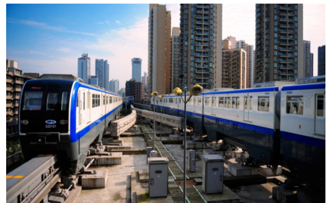
Fig. 6 Switch area of line 3 in Chongqing
