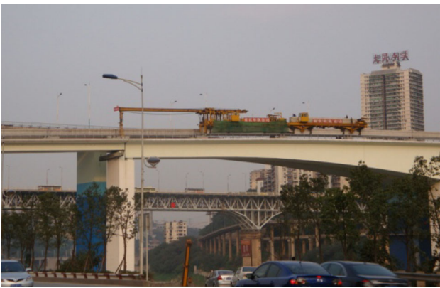
Fig. 15 Beam transport vehicle and erecting machine
