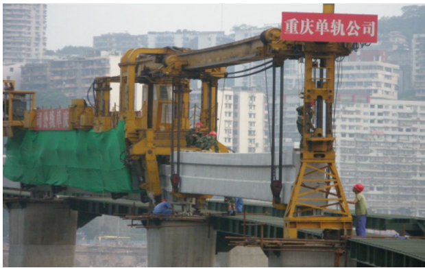
Fig. 14 All terrain, universal PC track beam erecting machine
