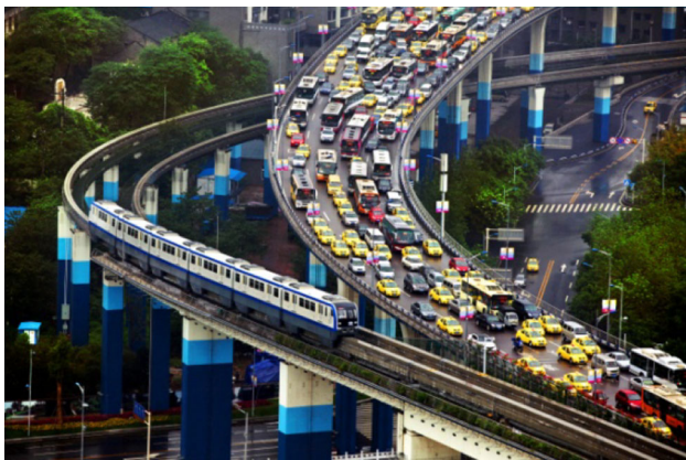
Fig. 10 Across Jialing River Bridge
