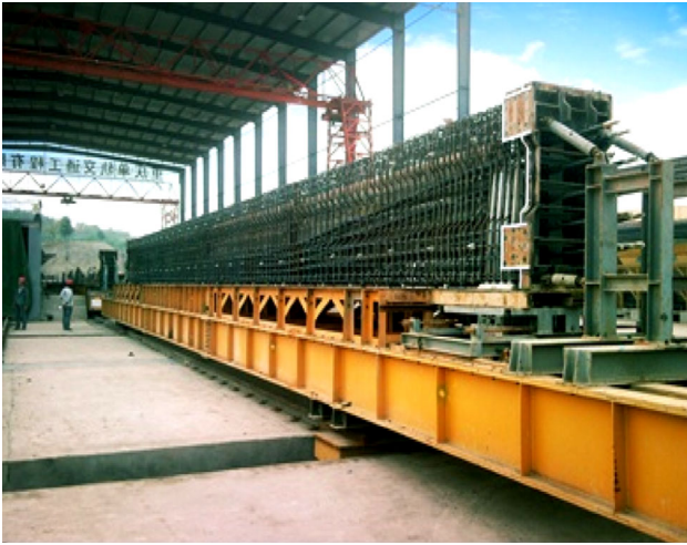
Fig. 13 Factory production of track beam
