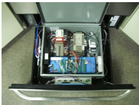
Fig. 3 The computer and the wiring as they were built for the first prototype
