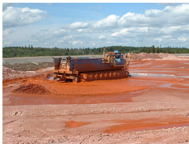
Fig. 6 Dry mud stacking
