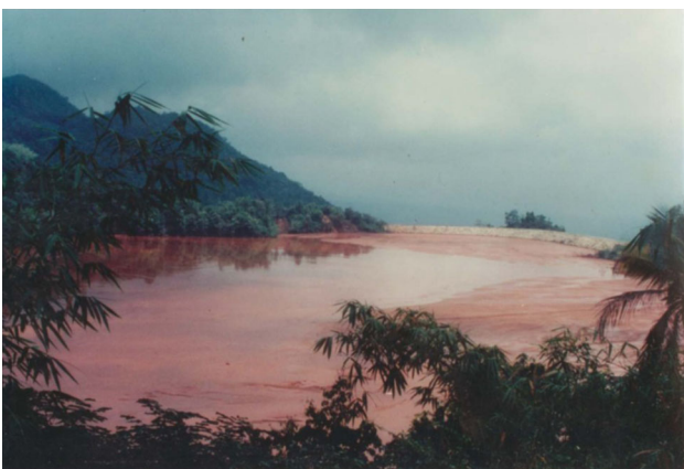
Fig. 3 Bauxite residue disposal into a dammed valley to create a lagoon, early stages, Mount Rosser, Jamaica
