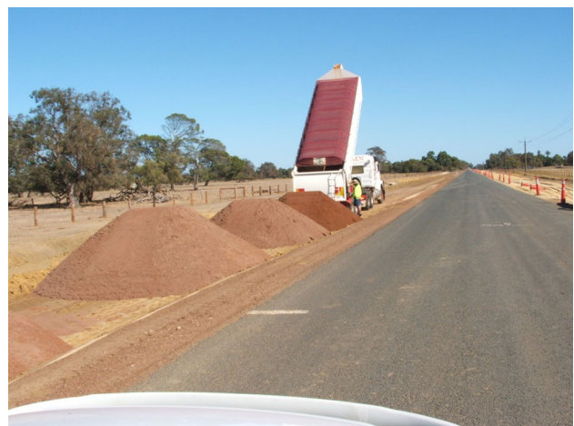
Fig. 12 Use of Red Sand™ for road construction (Photograph courtesy of Alcoa)
