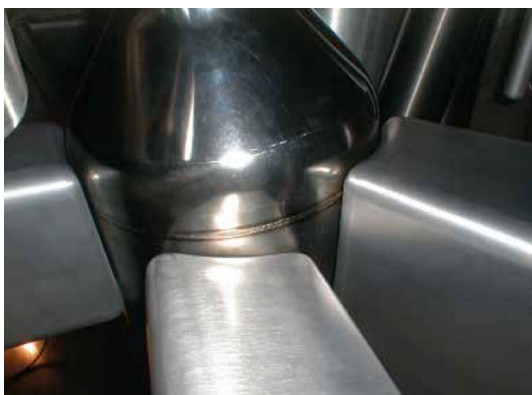
Fig. 16 Cold source vessel at the reactor FRM-II in Munich surrounded by three beam tubes [51]. In operation, the metal sphere in the middle contains 12 l of liquid deuterium at 18 K. Copyright Forschungsreaktor FRM II/Technische Universität München, reprinted with permission
