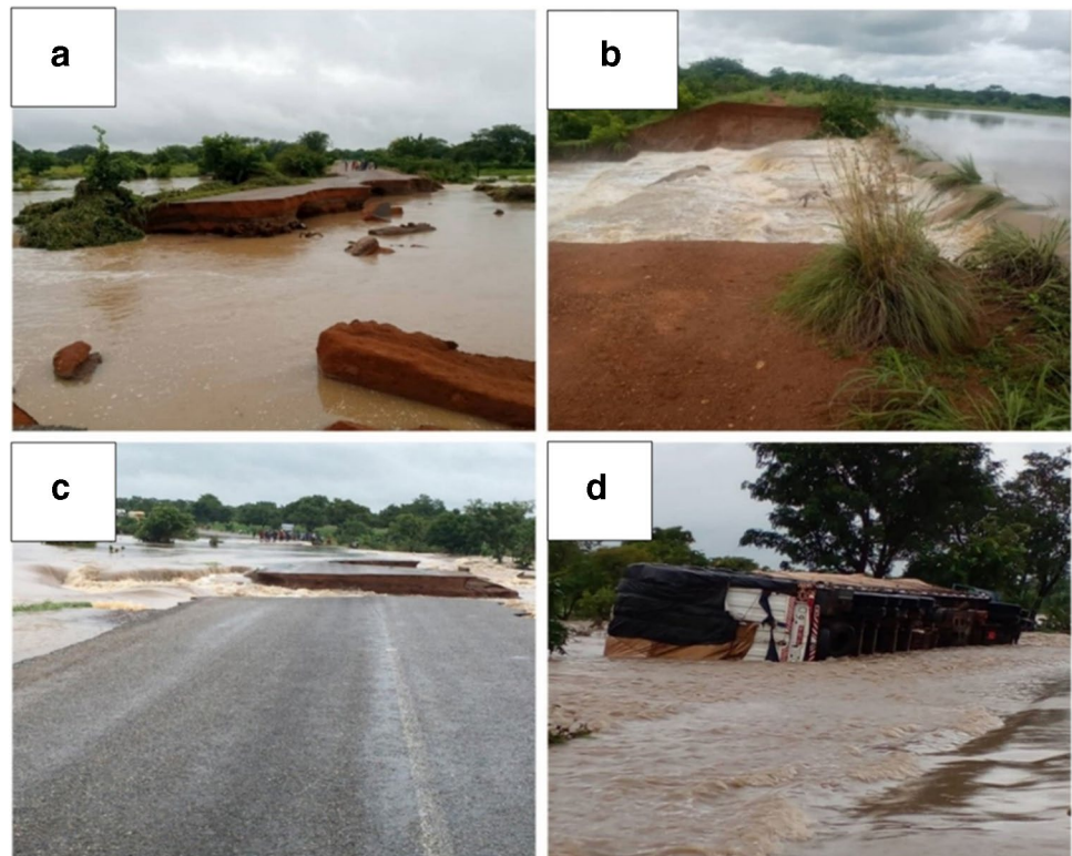
Fig. 1 Examples of flood disasters in 2021 in the region (a) Road washed off; b Daffiama-Sanwie Road; c Nadwoli –Wa Road; d Truck en route to Burkina Faso (Source: Ministry of Roads and Highways Ghana)
