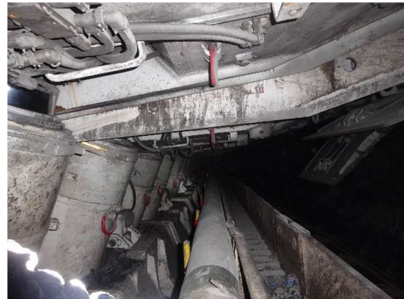
( a ) Hydraulic support crushed accident
