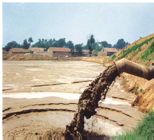
(c) Backfilling
