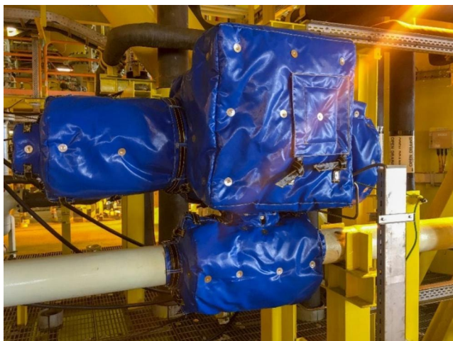
Fig. 1 An insulated actuated valve designed to conserve heat and protect personnel (Courtesy: Shutterstock)
