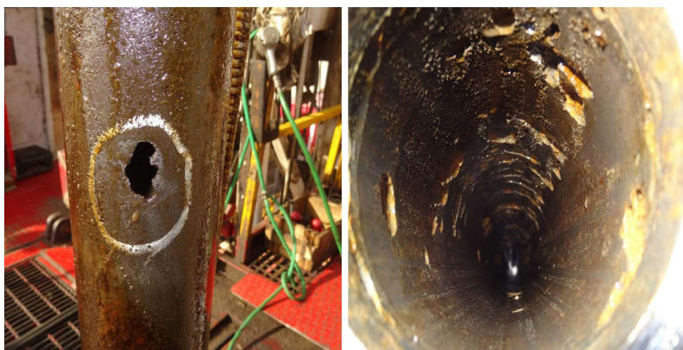
Fig. 2 Production tubing type (3 1/2 " 9.2, L80), an example of the impact of CO 2 corrosion leading to create holes
