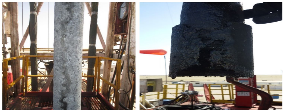
Fig. 5 Production tubing (2 7/8 in; N-80; 6.5 lb/ft), an example the effect of hydrogen corrosion on production tubing string
