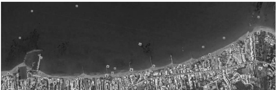
Fig. 8 Series of groins to protect from beach erosion downdrift of small port in Ag. Marina, Chania, Greece, Source: “Ag. Marina” 35°31′07.47” N and “23°55′09.03” E. Google Earth, April 18, 2015. July 2, 2015
