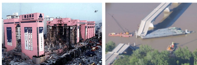
Fig. 1 Collapses of Sampoong Department Store, Korea (Left) and I-40 Mississippi River Bridge, U.S. (Right)
