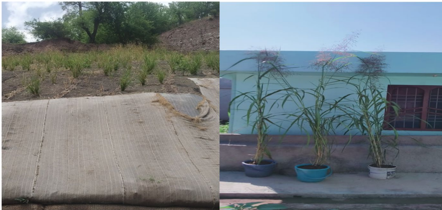
(b). The application of vetiver grass root in areas prone to landslides along roads.
