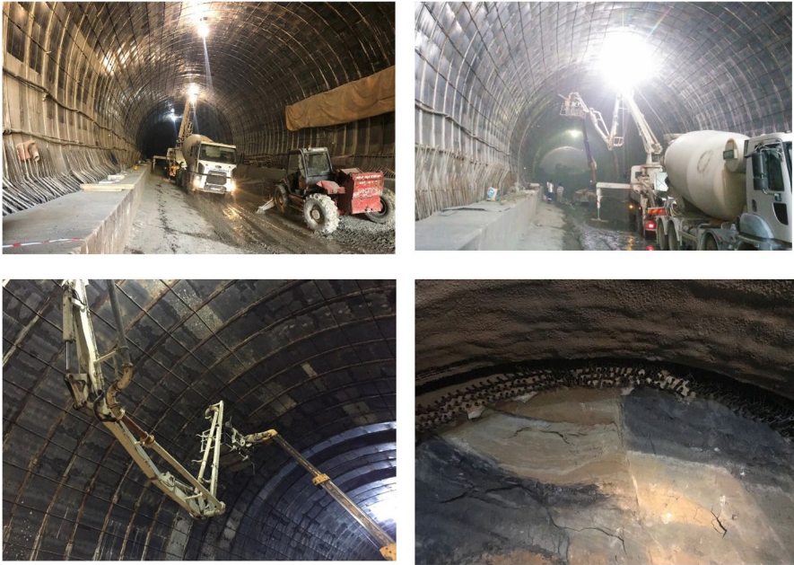
Fig. 30 Intermediate lining applications in the tunnel
