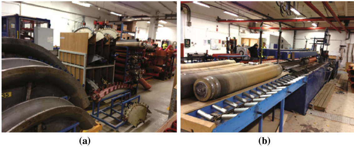
Fig. 3 Current pipe bending technology used in Pipelife Norge AS
