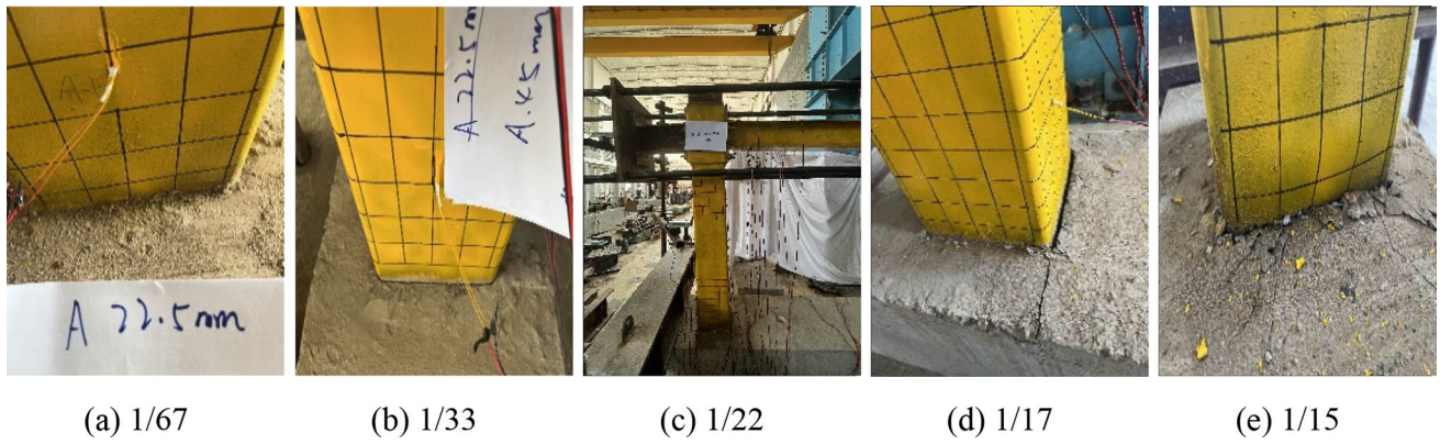
Fig. 12 The failure mode of the column under different horizontal drifts of the KJ-1
