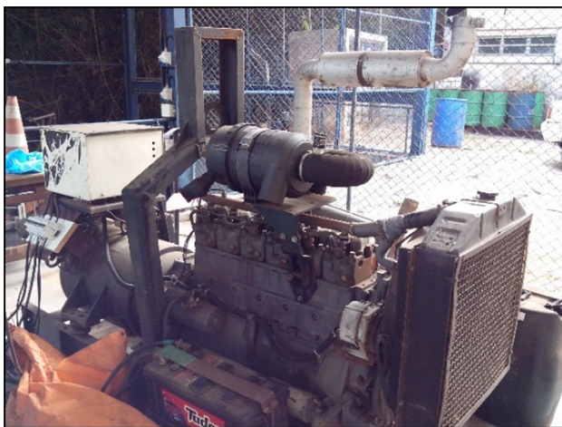
Fig. 1 Six-cylinder, four-stroke, MWM diesel engine
