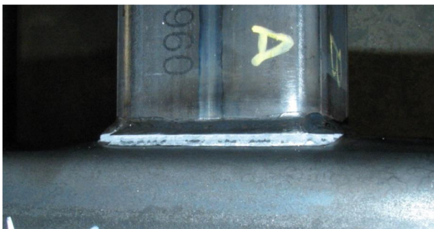
Fig. 2 Punching shear failure of a tubular X-joint made of UHSS
