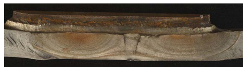
Fig. 16 Section through crack location 4 in specimen 3
