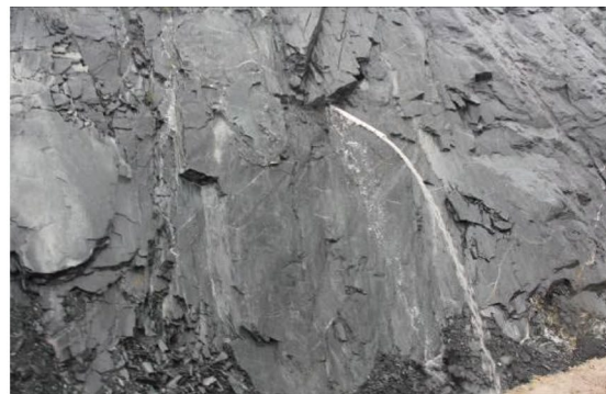
(b) Inclined drain holes
