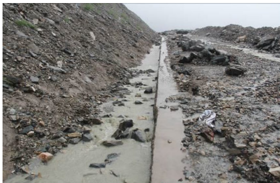
(a) Surface drainage ditch
