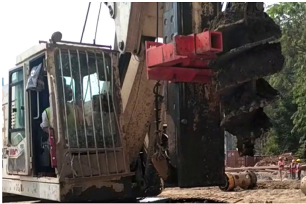
Fig. 11 Auger cleaner—during cleaning
