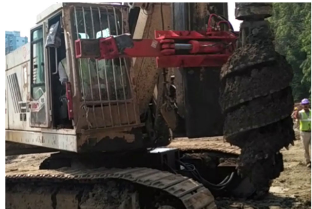
Fig. 10 Auger cleaner—during boring
