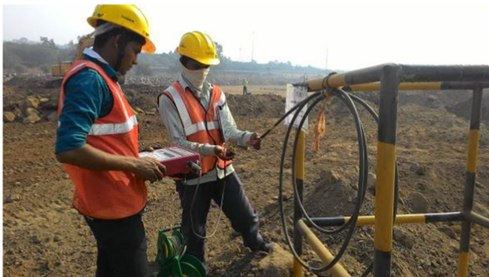
Fig. 20 Pore water measurements by vibrating wire piezometer
