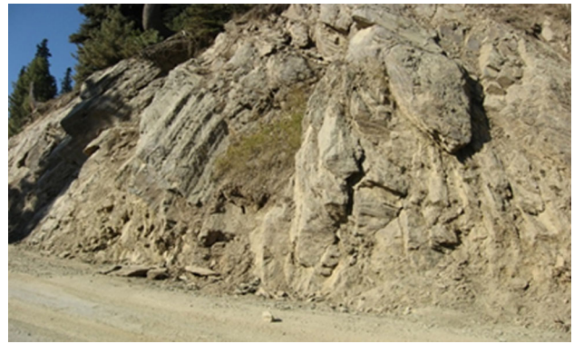
Fig. 39 Meta-siltstones of Halfkhalan formation showing excessive weathering close to surface
