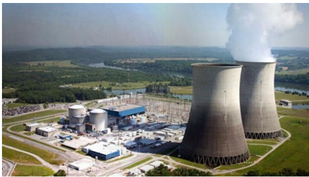
Fig. 25 Cooling towers in Kakrapar nuclear power plant [10]
