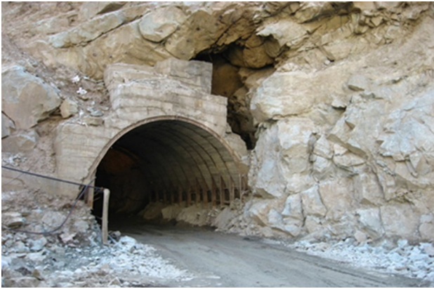
Fig. 37 Panjal volcanics exposed at diversion tunnel outlet
