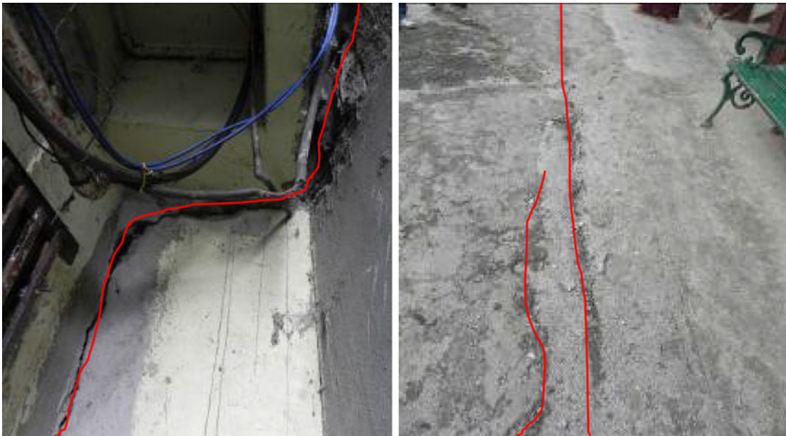
Fig. 9 Cracks (marked red ) on the road due to creep of soil in Gangtok. (Color figure online)
