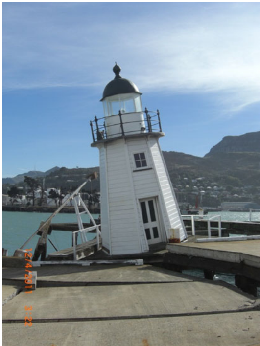
Fig. 1 Damage to a historic light house at Lyttleton port
