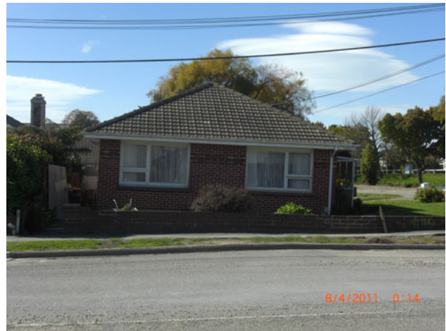
Fig. 3 Settlement and rigid body rotation of a house following soil liquefaction
