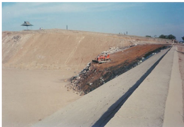
Fig. 7 Waste filling at Ankleshwar Landfill
