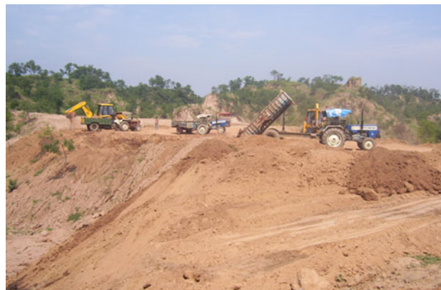
Fig. 15 Earth filling operations
