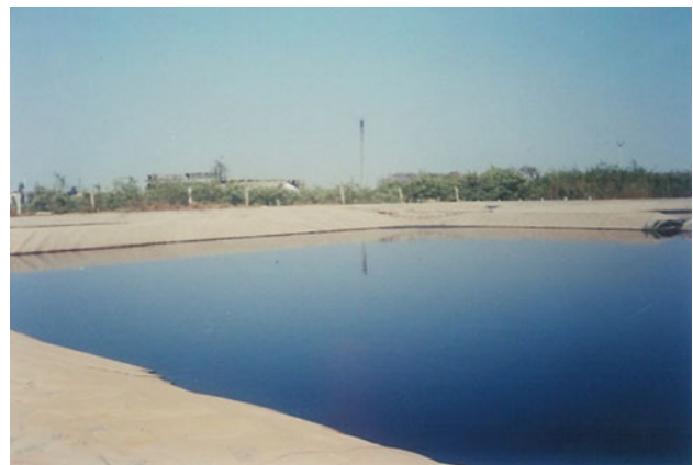
Fig. 12 Leachate solar pond
