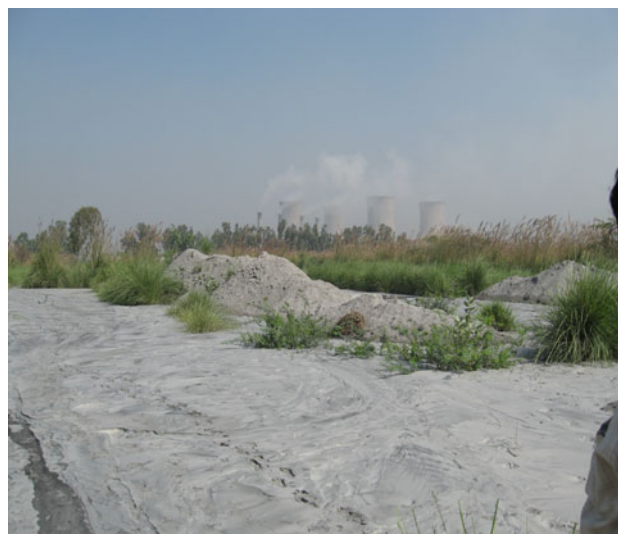
Fig. 32 View of ash pond
