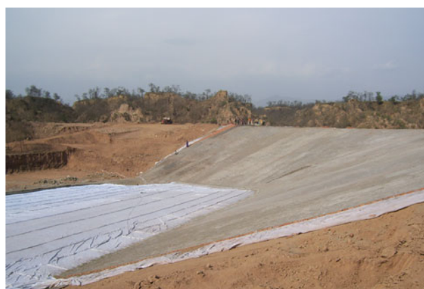
Fig. 16 Completed phase of landfill
