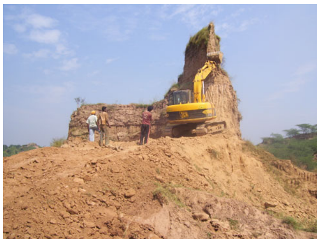
Fig. 14 Excavation of earth mounds
