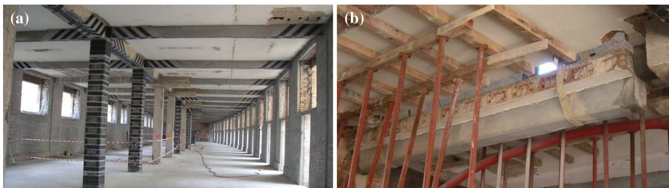
Fig. 1 Retrofitting of the RC building (a) and removal of the beams (b)
