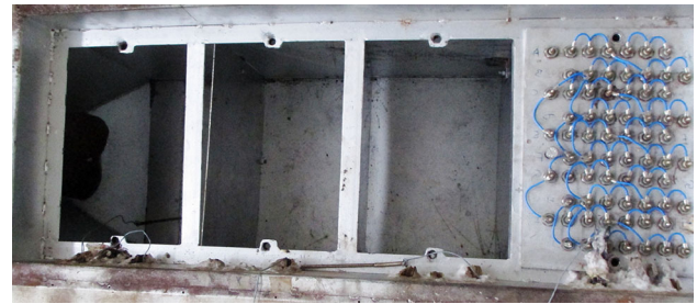
Fig. 2 Photograph of heater bank with baffles
