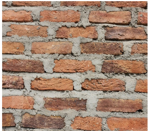
Fig. 2 Typical thickness of vertical joint and mortar layers in burnt clay bricks masonry
