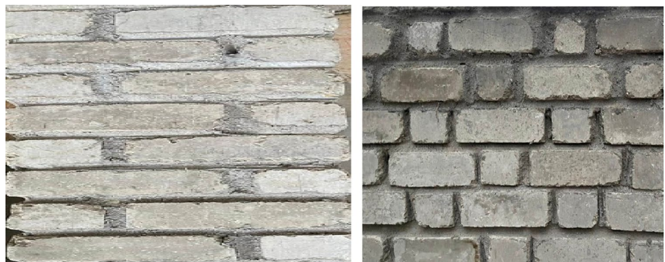
Fig. 2 Typical thickness of vertical joint and mortar layers in burnt clay bricks masonry
