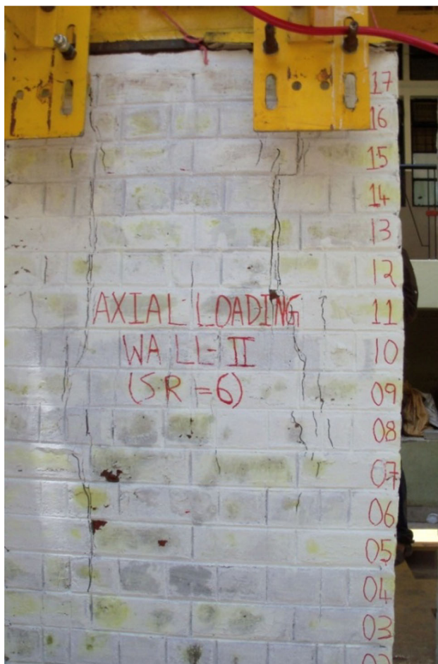
Fig. 5 Typical vertical cracks in TMB-225-A-2
